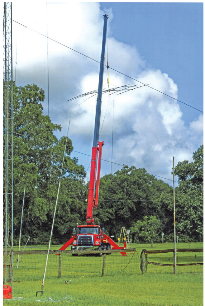
Being without a tower didn't stop the Sun Country Amateur Radio Society, KB4KP, in Marion County, Florida, from operating in the 2021 ARRL Field Day. Instead, they suspended one of their antennas from a crane brought in specifically for the event. The crane was secured in a fenced-in area that was adjacent to their three operating positions. [Bruce Richardson, WA4IPU, photo]
